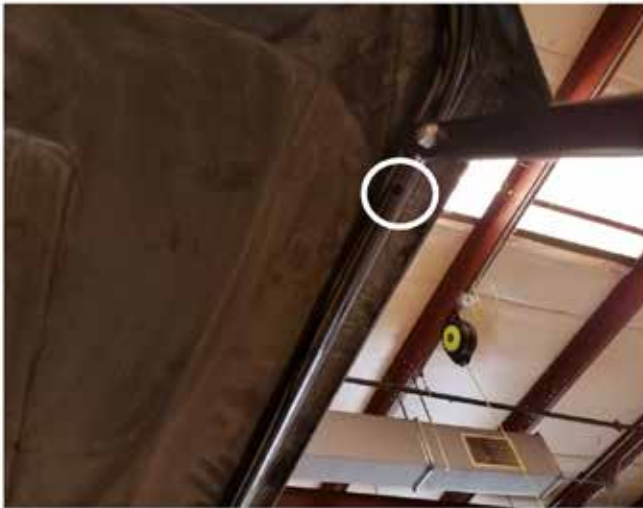
54. Place the roof on top of the roof hoop and line up the 4 holes.
