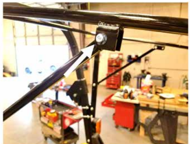
14. On the "passenger" (right) side, attach stay rod (#4) to roof hoop bracket in the hole using m8x40 flange bolt as shown. Button head must be facing outward to avoid interference with textile panel.
